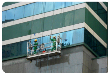
High-Rise Roof & Structural Cleaning Services
